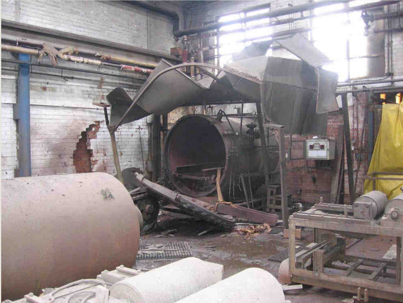
Failed Rubber Autoclave
